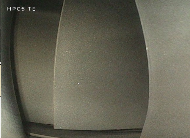
STAGE 5 HPC: SEVERAL HPC5 LE BLADES OBSERVED WITH MINOR DENTS TO LE IN LOWER 25%, DIM B & DIM A. ALL WITHIN AMM LIMITS. SERVICEABLE - NO LIMITATIONS
